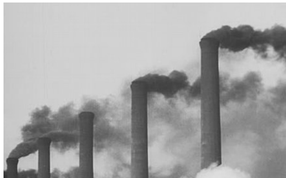
Figure 5. 1 Downwash as a result of unstable conditions.
