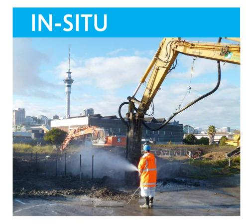
Application via a water blaster during the in-situ trial due to the coincidental emission of cement dust.
