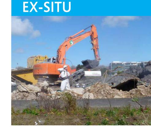
Backpack mist blower used during the ex-situ trial due to reduced dust emission.
