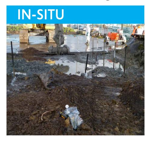
Concentrations reduced by approximately a factor of ten between the source and receptors located some 10m away from the trial work area.
